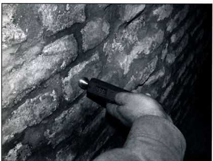
■ Photo 6-7. Salt crystallization during the reconstruction at Véstő-Mágor
